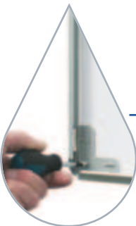
Fix in place.
